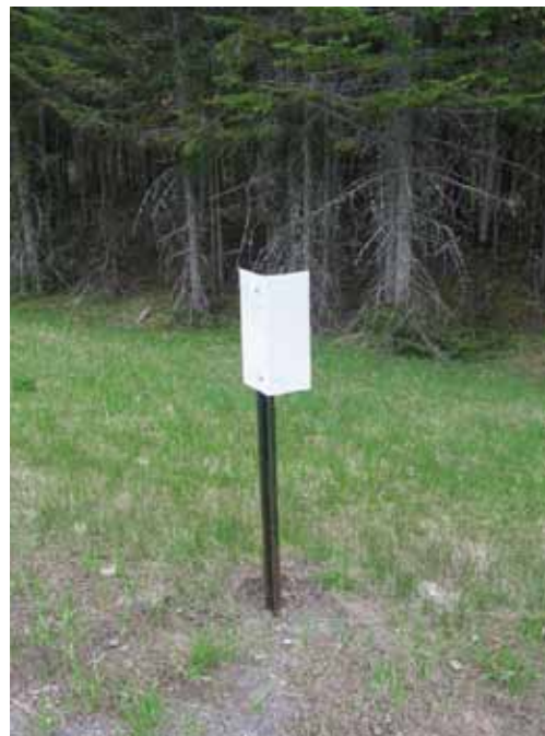
Reflector detail MaineDOT photo- Richard Bostwick
